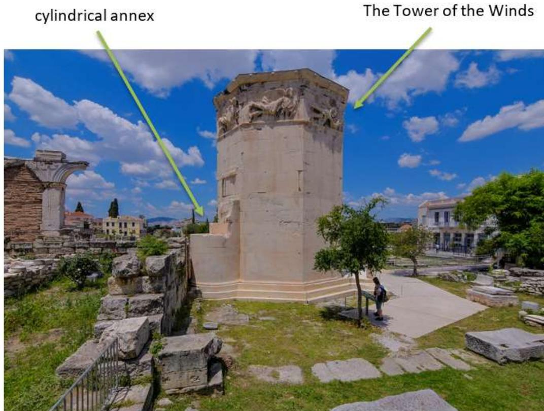
**Fig. 7.** The Roman Agora in Athens viewed from the SE, showing the cylindrical annex attached to the main octagonal building of the Tower of the Winds. The arched lintels (see also Fig. 1) connected to the Agranomeion building complex are visible on the left. Photo © PAPADIMITRIOU
