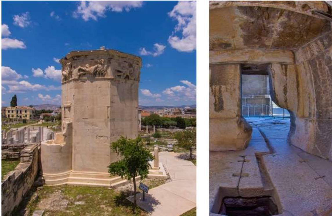
**Fig. 4.** Views of the exterior (left) and interior (right) of the cylindrical annex from the E and S respectively. The opening in the interior leads to the inside of the octagonal building. Straight channels on the floor carry water to the inner part of the building (see Fig. 5). Photos © PAPADIMITRIOU
